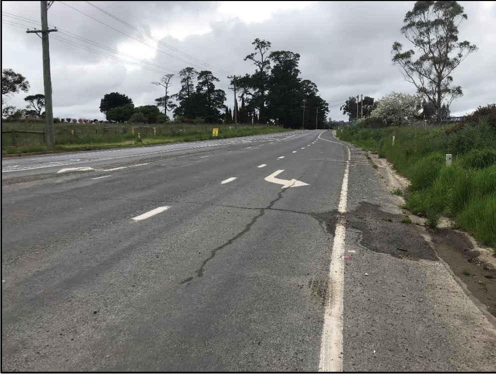
Photo 4 – Existing left turn deceleration lane for traffic turning off Berrima Road into Bowman Road
